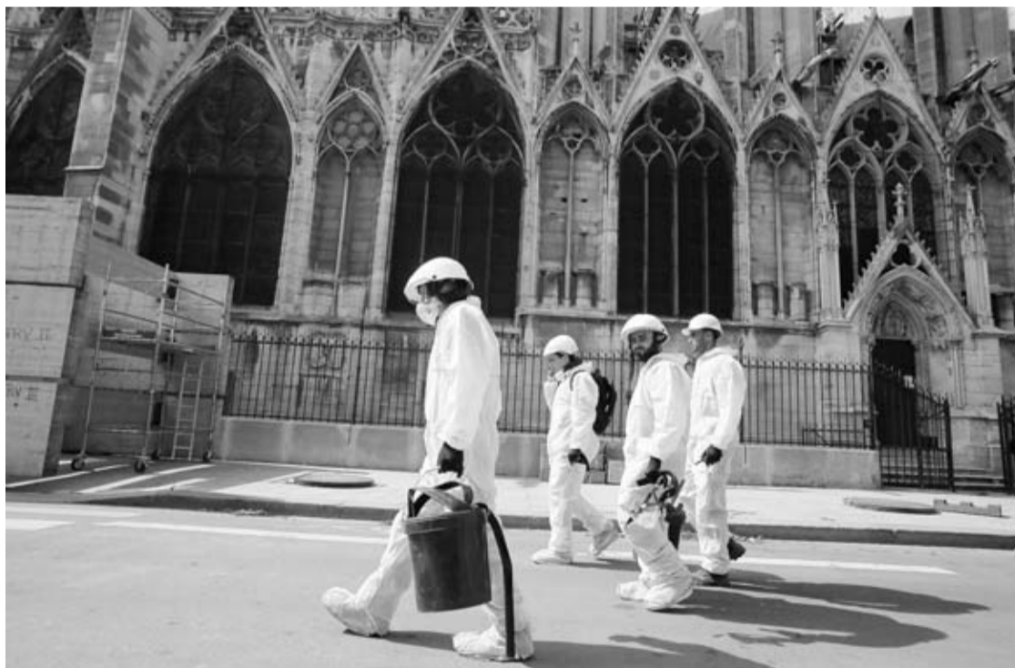
Workers dressed in white overalls walk past the Notre Dame Cathedral, in Paris, Thursday, Aug. 1, 2019, as the preliminary work begins to repair the fire damage.
